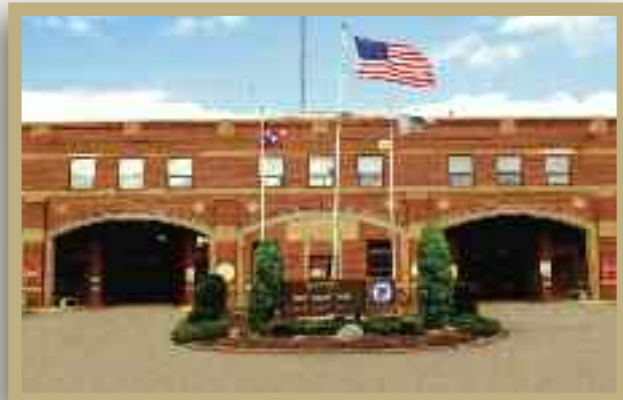
Water Distribution Johnston Street, Akron, Ohio
