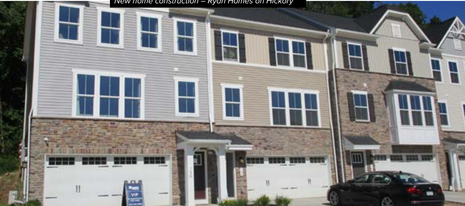
New home construction – Ryan Homes on Hickory
